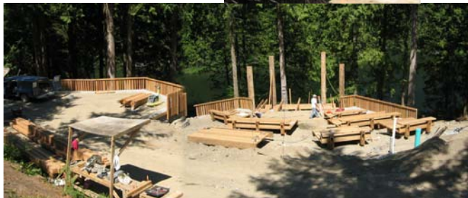
The Loon Lake Amphitheatre under construction
