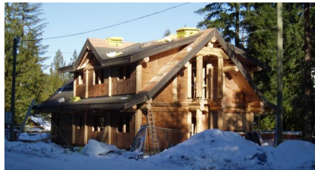
The new cabins for Loon Lake take shape – December 2007
