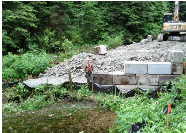
Construction of the Spring Creek Bridge and gas-line crossing
